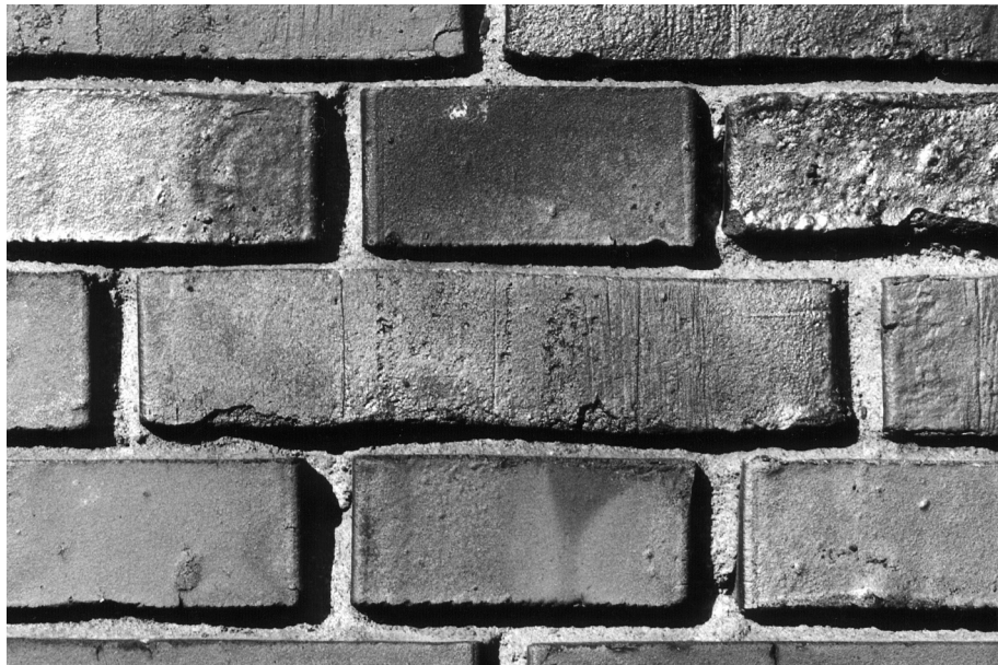
4. The wall's 'clinker' bricks
